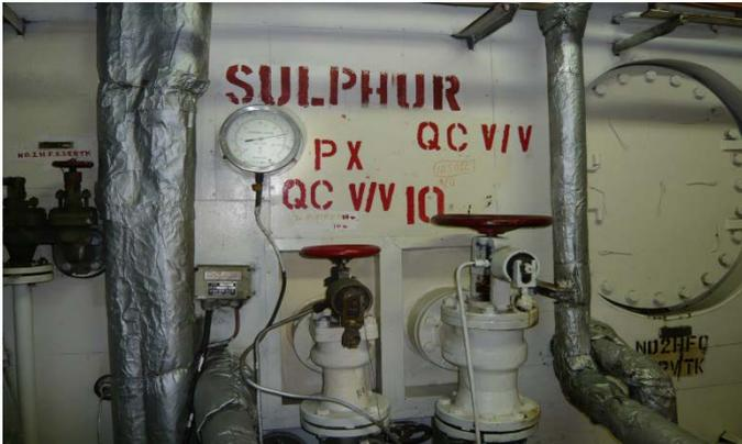
In 2011 the United States Coast Guard (USCG) published a [Safety Alert](#) regarding the inspection of fuel oil quick-closing valves. The safety alert was issued after Port State Control (PSC) officers found that fuel oil tank quick closing valves had sometimes been blocked in an open position, or were poorly maintained so that they were not operating as designed when released in an emergency. It would appear that this is still an ongoing issue.
